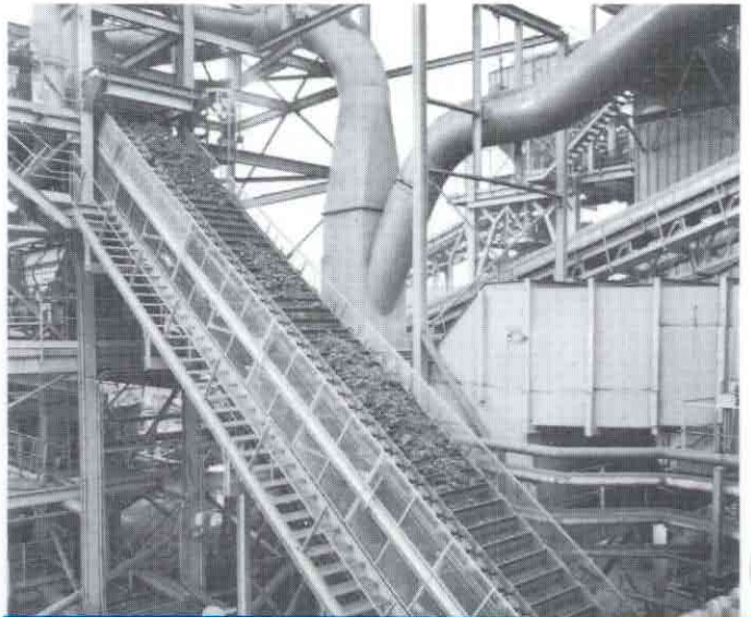
Rex apron conveyor handling hot sinter in this steel mill.
